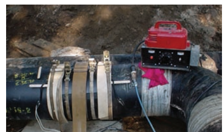
PTJC with Straps and Fusion Welder
